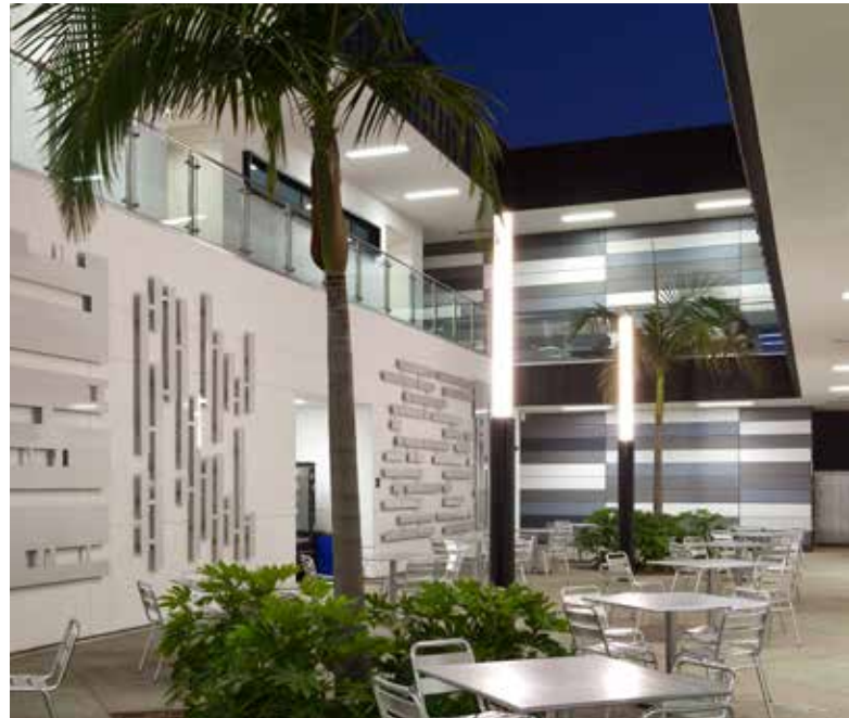
San Diego Community College North City Campus - San Diego, CA Architect: Joseph Wong Associates JWDA | Photography: Balfour Beatty Construction
