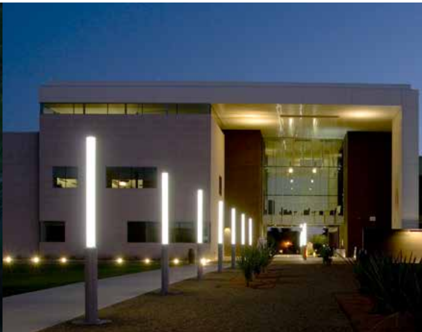
CNM Student Resource Center - Albuquerque, NM Architect: AECOM Design | Photography: David Nufer Photography
