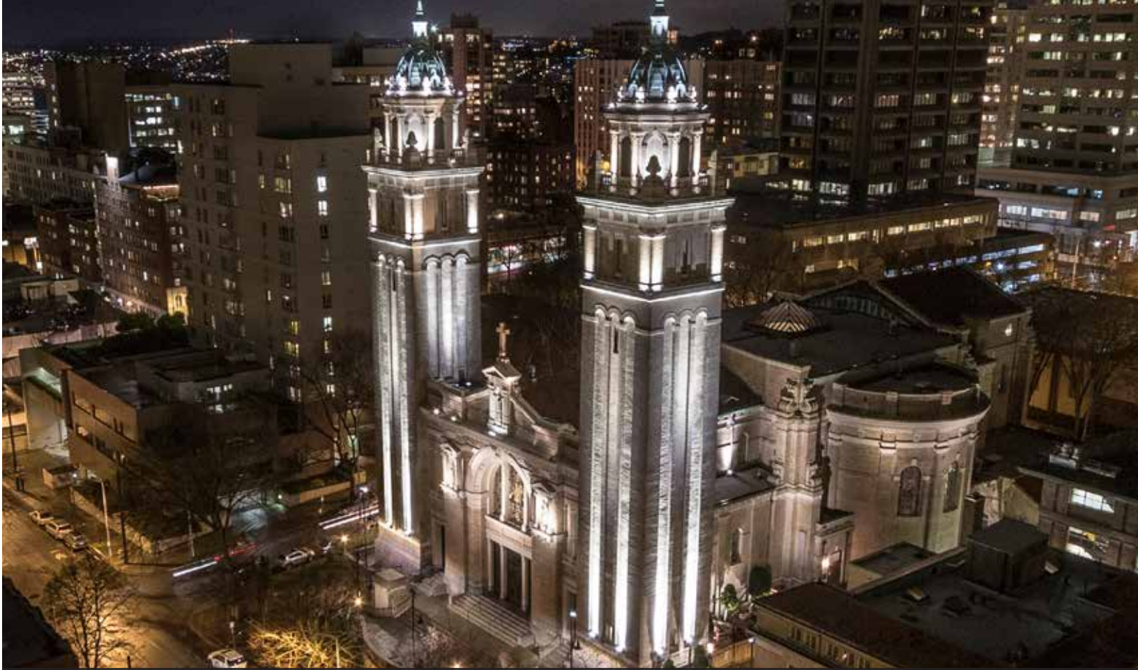
St James Cathedral - Seattle, WA Lighting Designer: Linet Henry of Eluned Lighting | Photography: Tom Reese
