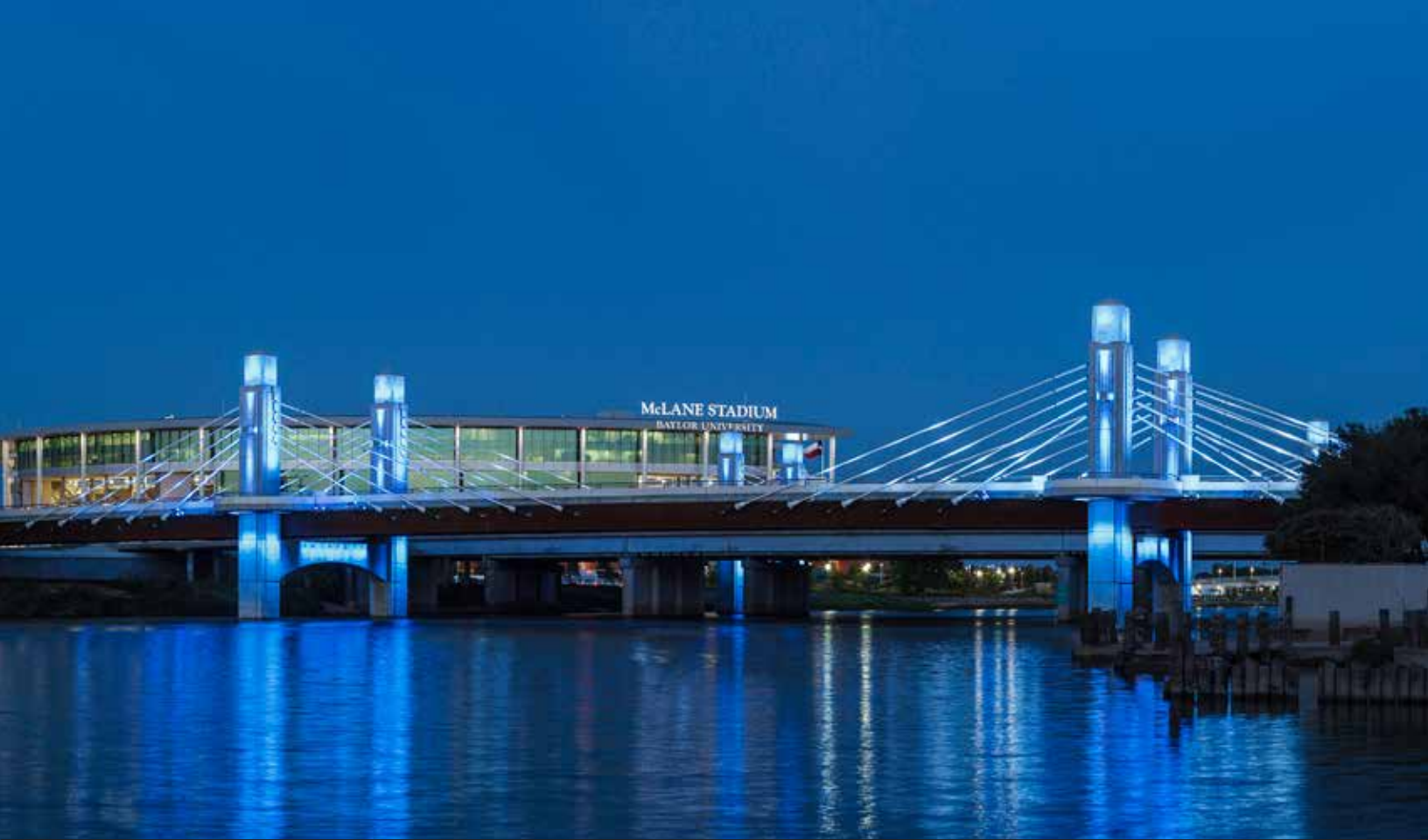
I-35 Brazos Bridge - Waco, TX Engineer: Finely Engineering Group | Photography: Joe Griffin Photography
