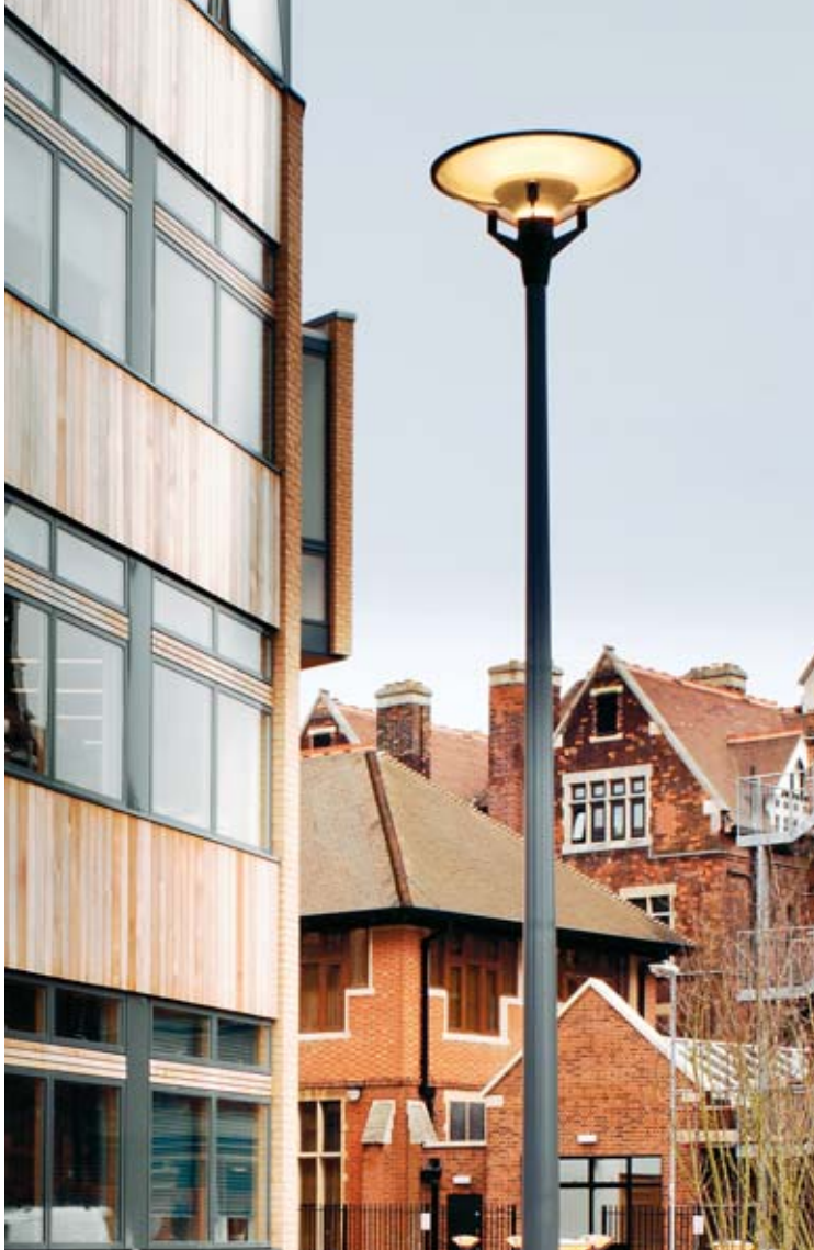
The Kipp outdoor fixture provides general lighting at the front of the building and announces the transition to the city of Cambridge.
