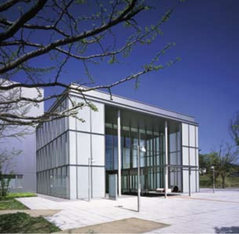
Opalised glass has been used at the entrance to provide diffuse light to the eight storey high hallway.
