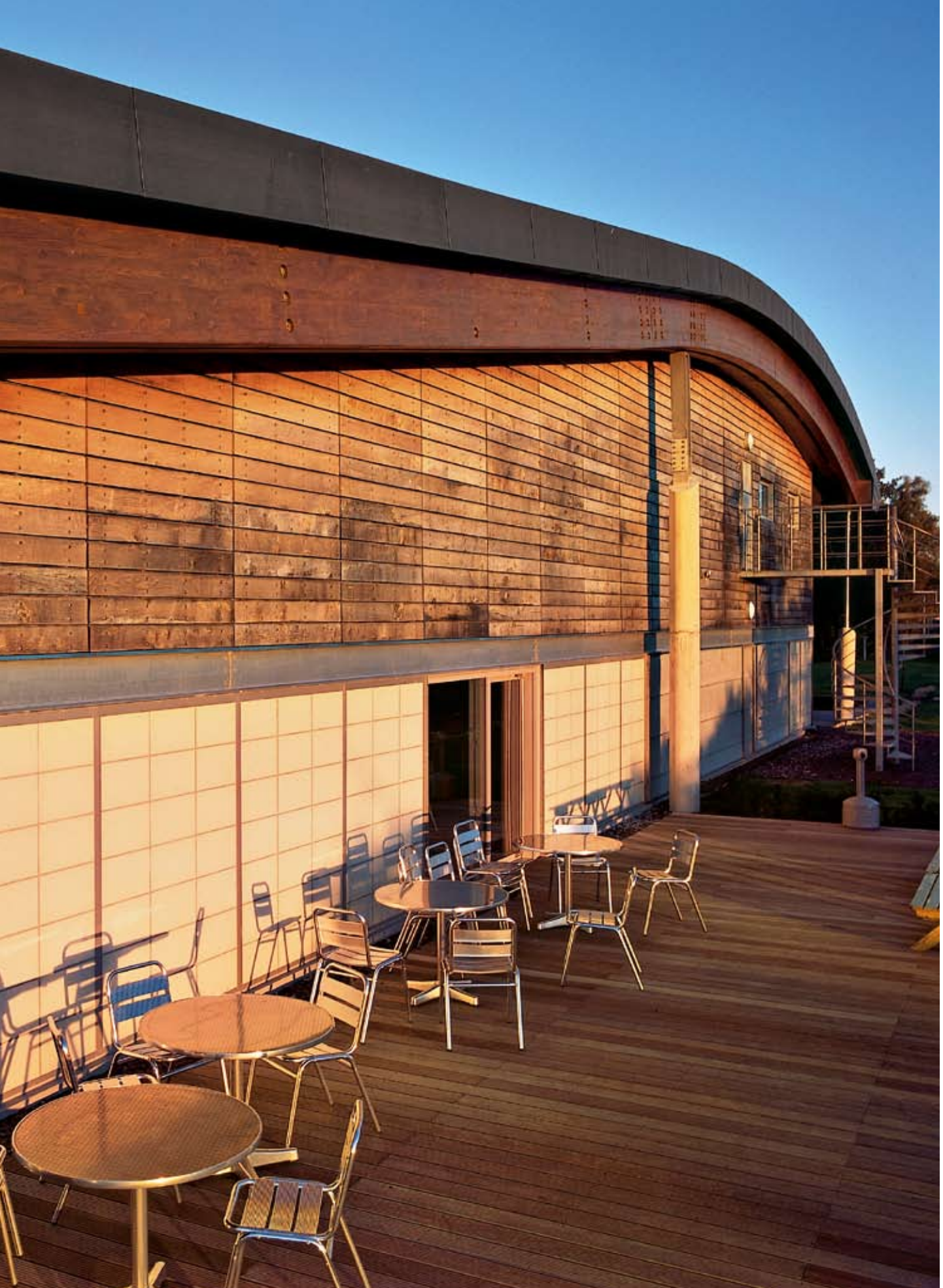
The ground floor façade consists of fibre glass sandwich panels that transmit light well. During the day, the opal material lets masses of daylight into the building. In the evenings, the illuminated elements appear to make the building hover above the dark landscape.
