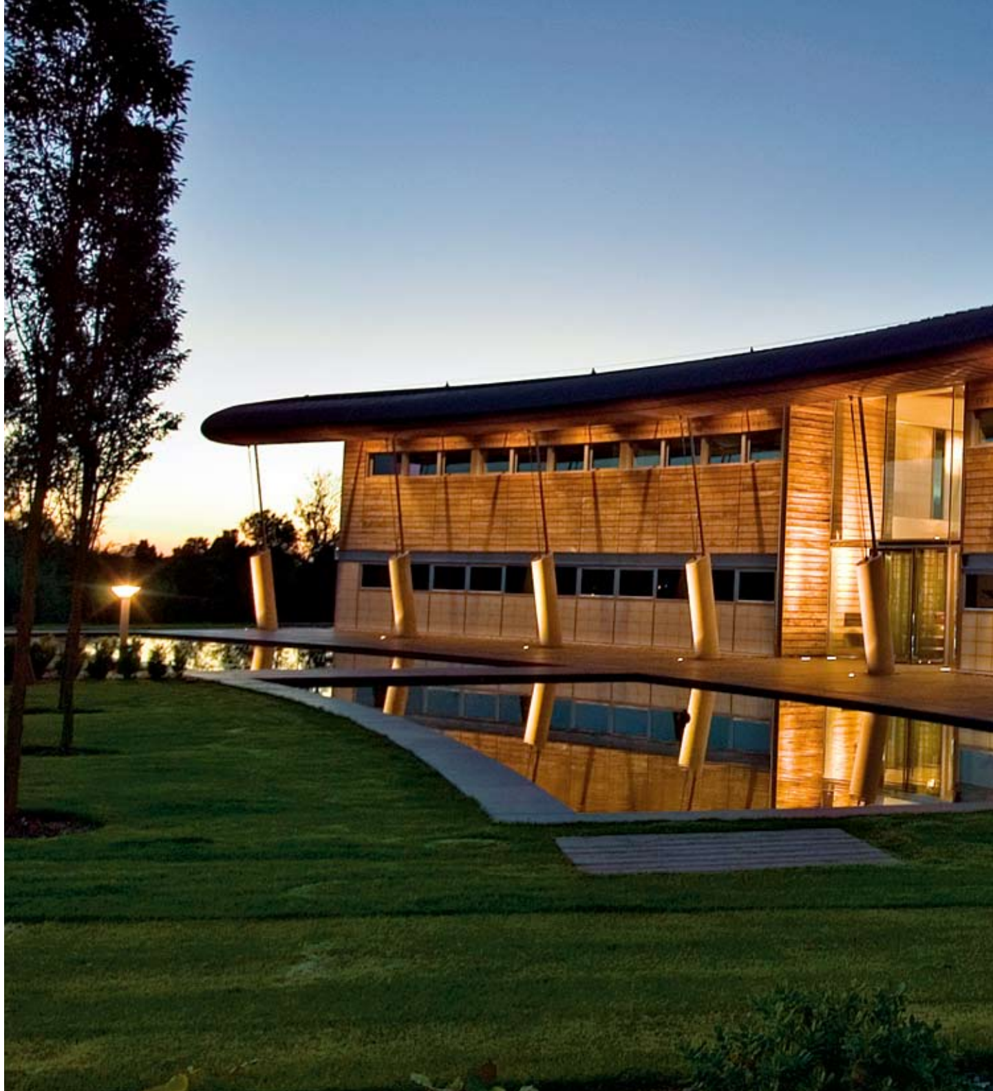
The most striking feature is the big, wave-shaped roof, which is supported by pairs of 44-metre long laminated wood beams stretching across the breadth of the building.
